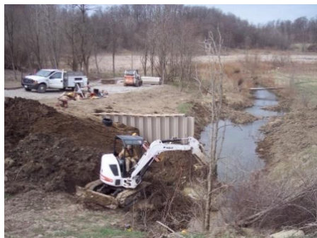
Fig 9. Construction of ditch plug for wetland restoration. (Photo: USFWS)
