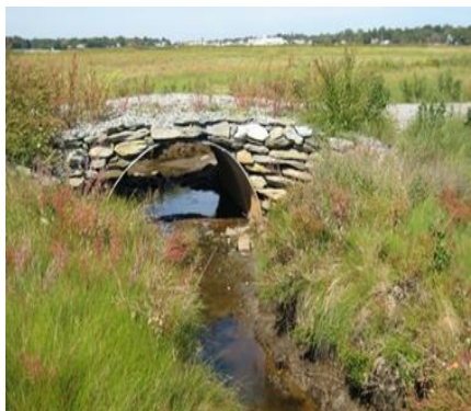
Fig 2. Culvert installed following restoration of a salt marsh at Jacob's Point, Narragansett Bay, Rhode Island. (Photo: Save the Bay )
