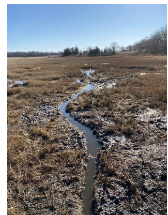
Fig 10. A hand-dug runnel drains excess water to restore tidal hydrology. (Besterman et al. (2021)
