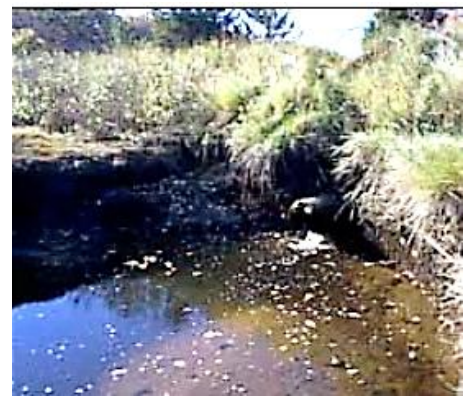
Fig 3. Culvert sited too high in the bank to allow for full tidal range. (Photo: Cape Cod Commission, 2001 )
