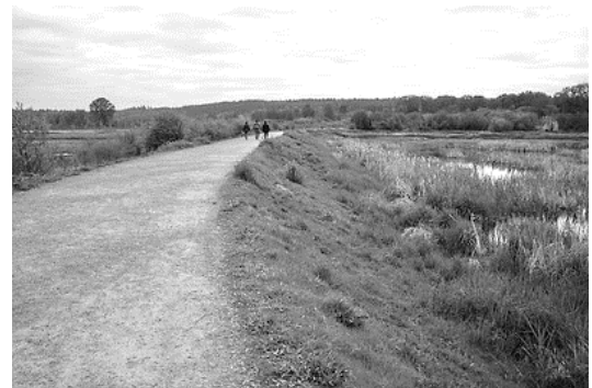
Fig 5. Example of dike built to drain a salt marsh for farmland (Photo: Isen Sno)
